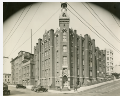
Cooper Medical College Building with Addition of 1890
